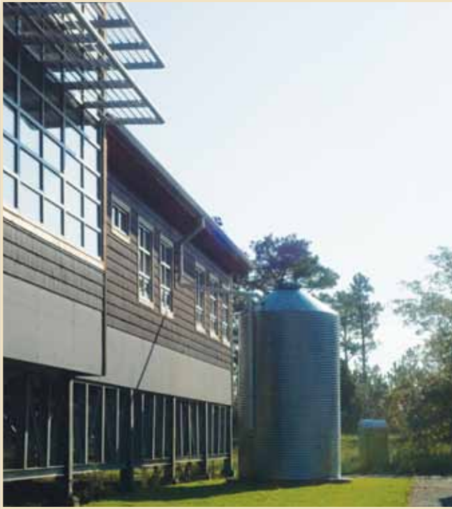
South side of building with rainwater collection cistern
