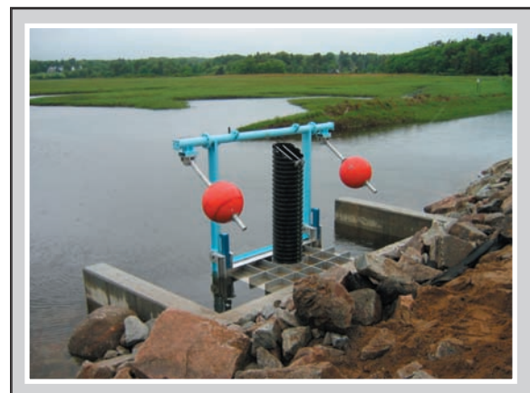
New box culvert and self-regulating tide gate at Drakes Island Marsh, near the Wells NERR.
